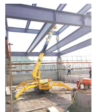
installation of steel structure of workshop
