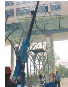
installation of glass
